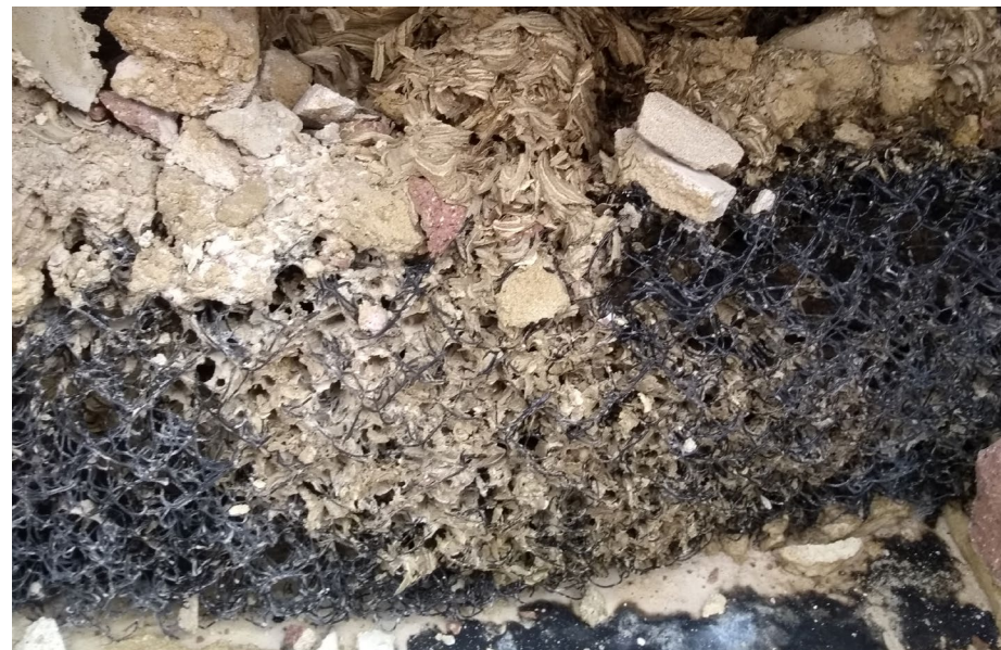
Single level mortar net.
