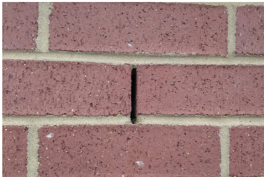
Mortar left out of joint, but plastic weep not installed.
