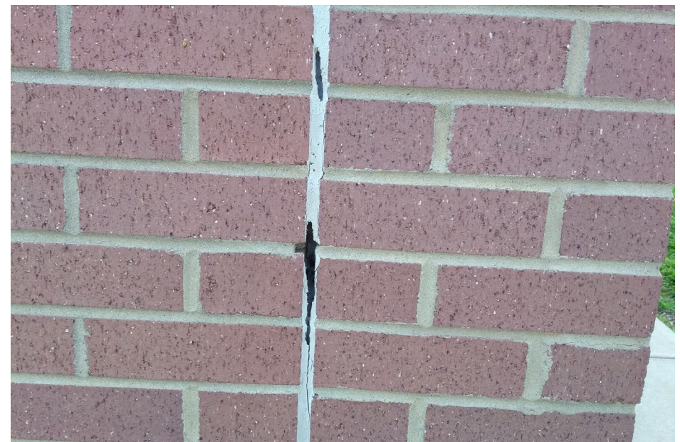
Failed sealant in expansion joint. (West wall)
