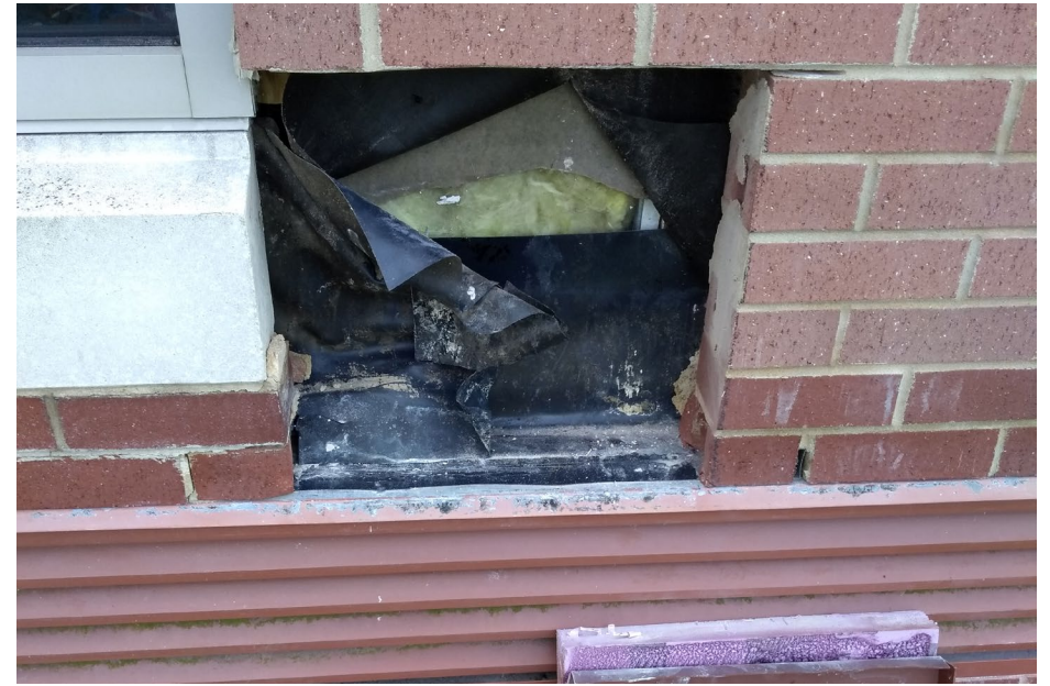
Insulation exposed because sheathing does not extend to bottom of wall. (Probe 5)
