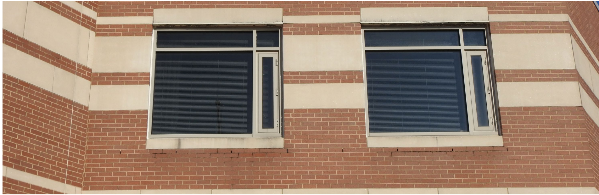
Dark biological staining under windows showing possible water infiltration areas.
