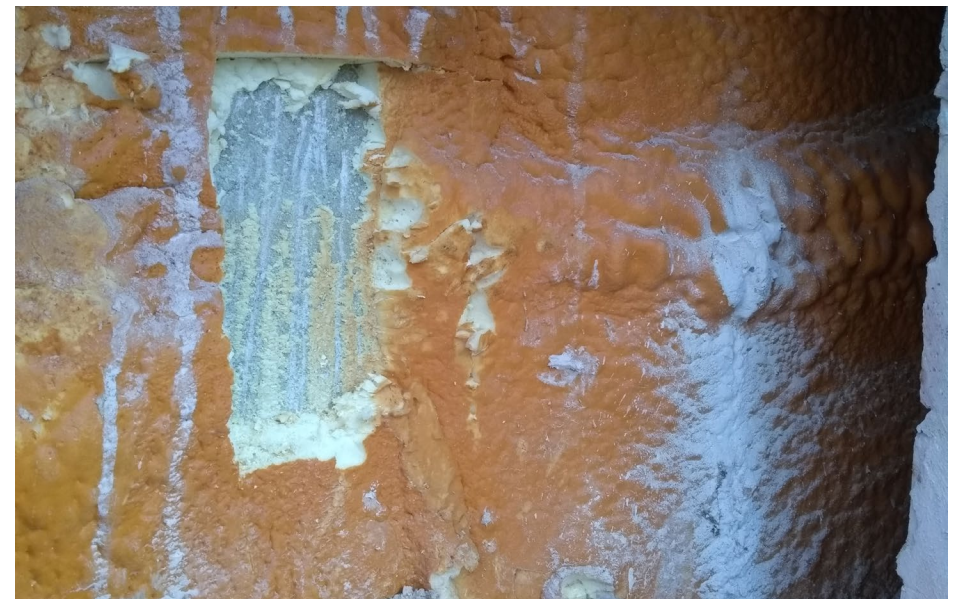
Spray foam insulation less than 1/2" thick. (Probe 18)
