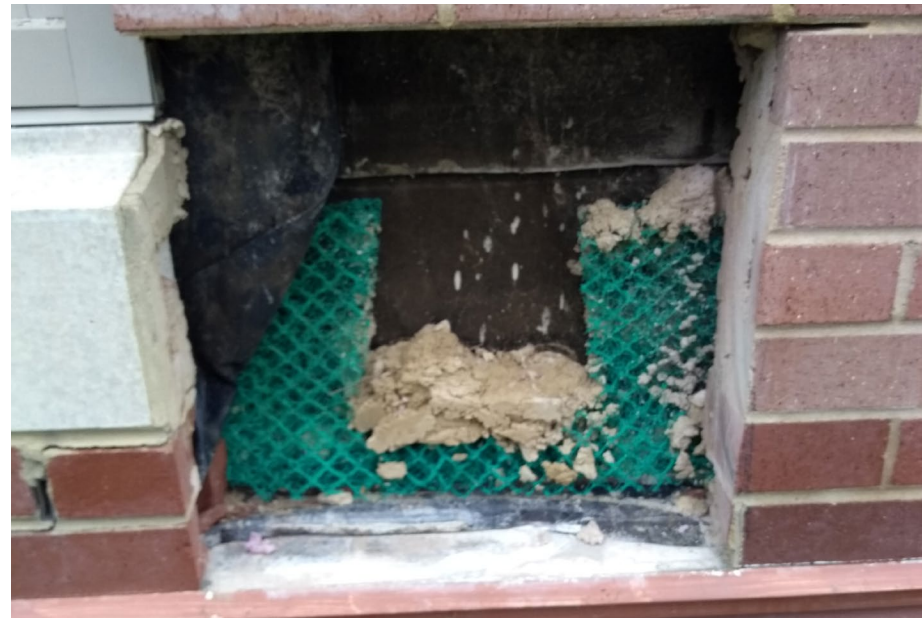
Dual level mortar net.
