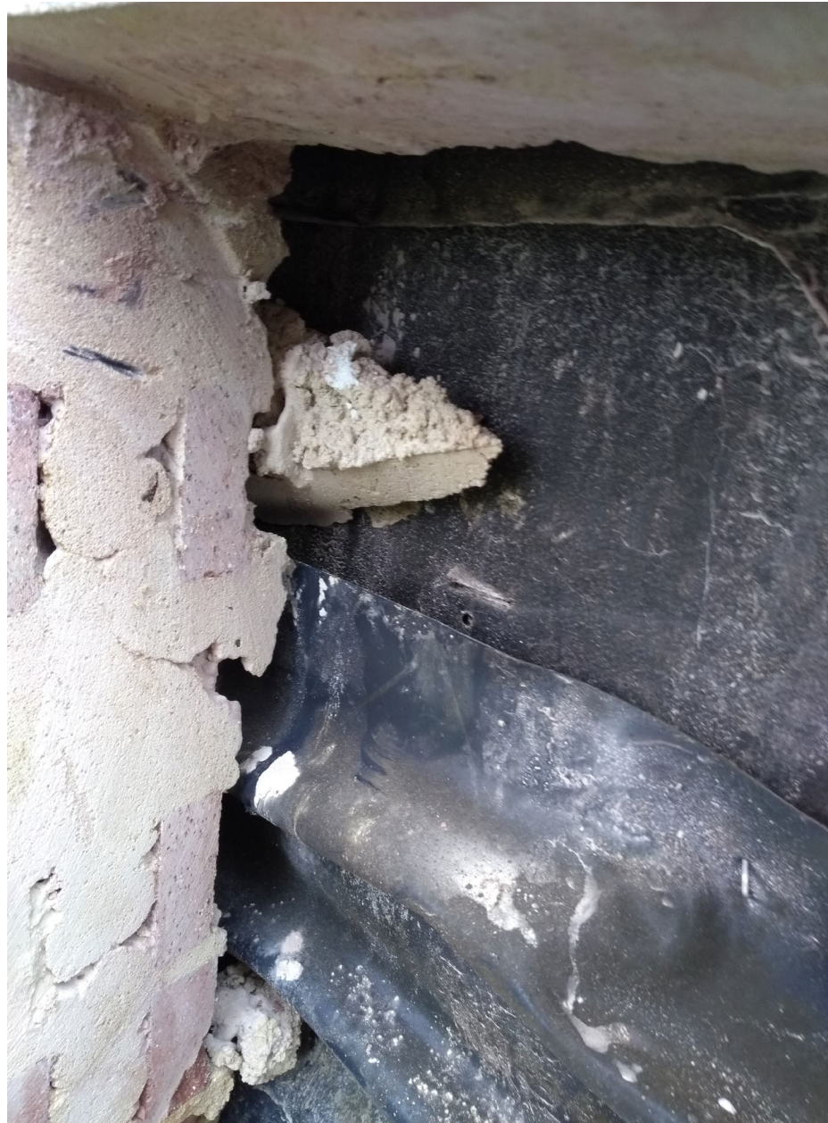
Flashing loose laid in wall with anchoring at the top. Does not direct water out of wall.
