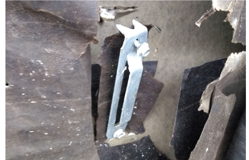
Masonry tie not secured into structural wall.
